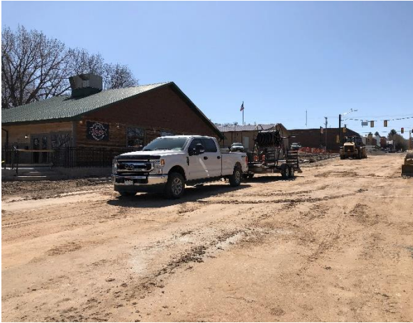
Installing last conduit from Hwy. 34 to 2nd Street on east side
