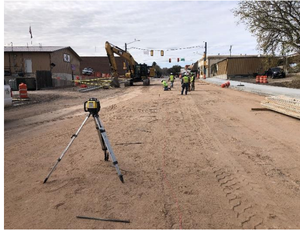
Final grading of west road sub-grade from Hwy. 34 to 2nd Street.
