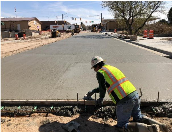
Concrete placement west center lane north of Highway 34
