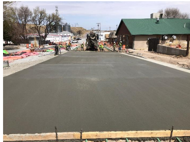
Concrete placement east center lane north of Highway 34
