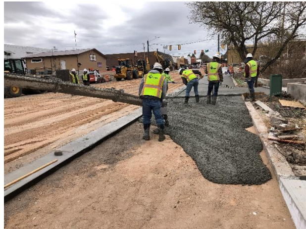
Concrete placement east sidewalk north of Highway 34 adjacent to pavilion.
