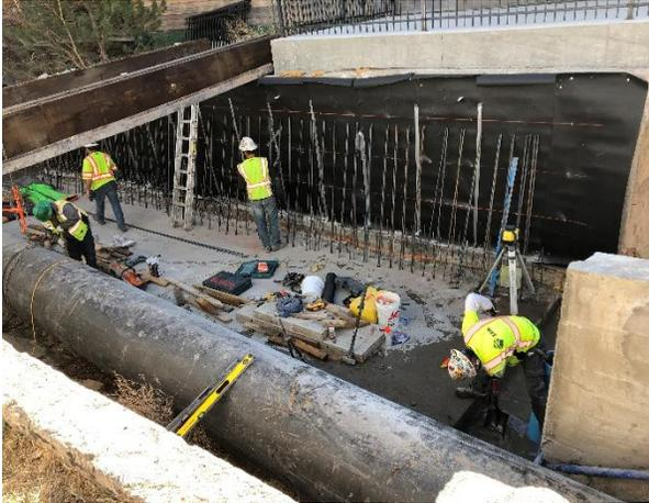
Construction of rebar wall cage adjacent to The Boonies
