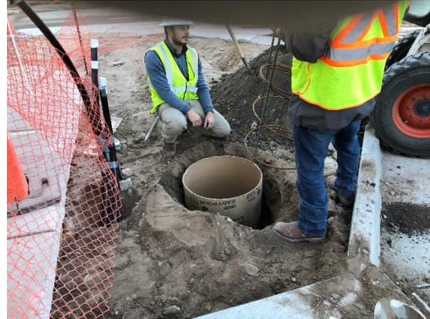
4D Electric installing 24"x48" sonotube base for light pole
